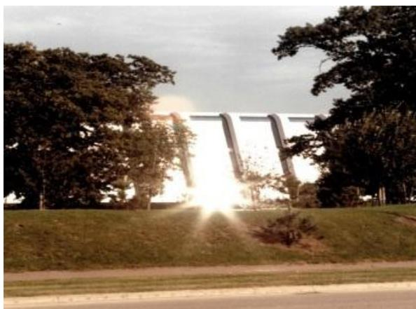
The photo to the left shows reflection of sunlight at the bottom of a sloping façade. The sun was high in the sky when the picture was taken. Flat facades reflect the sun without concentrating it. Facades which are concave can focus the sunlight and create areas of concentrated solar radiation. A separate Planning Advice Note 'Solar Convergence' gives advice on this issue.
