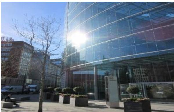
When the sun reaches the building at a glancing angle, more of it is reflected. For clear double glazing, the reflectance rises to 15% if the sun is at 45 degrees to the glazing, 22% at 60 degrees, and 49% at 75 degrees. Glare also depends on the angle of the sun and the angle at which the building is viewed.
